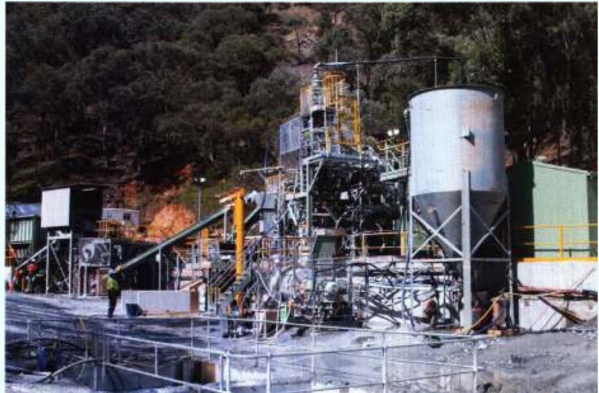
Hill End 120 tpd gravity plant.
